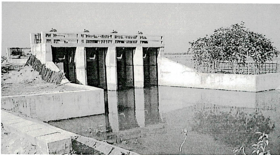
4 Vent Regulator, Chir Chir Chara Sub project
