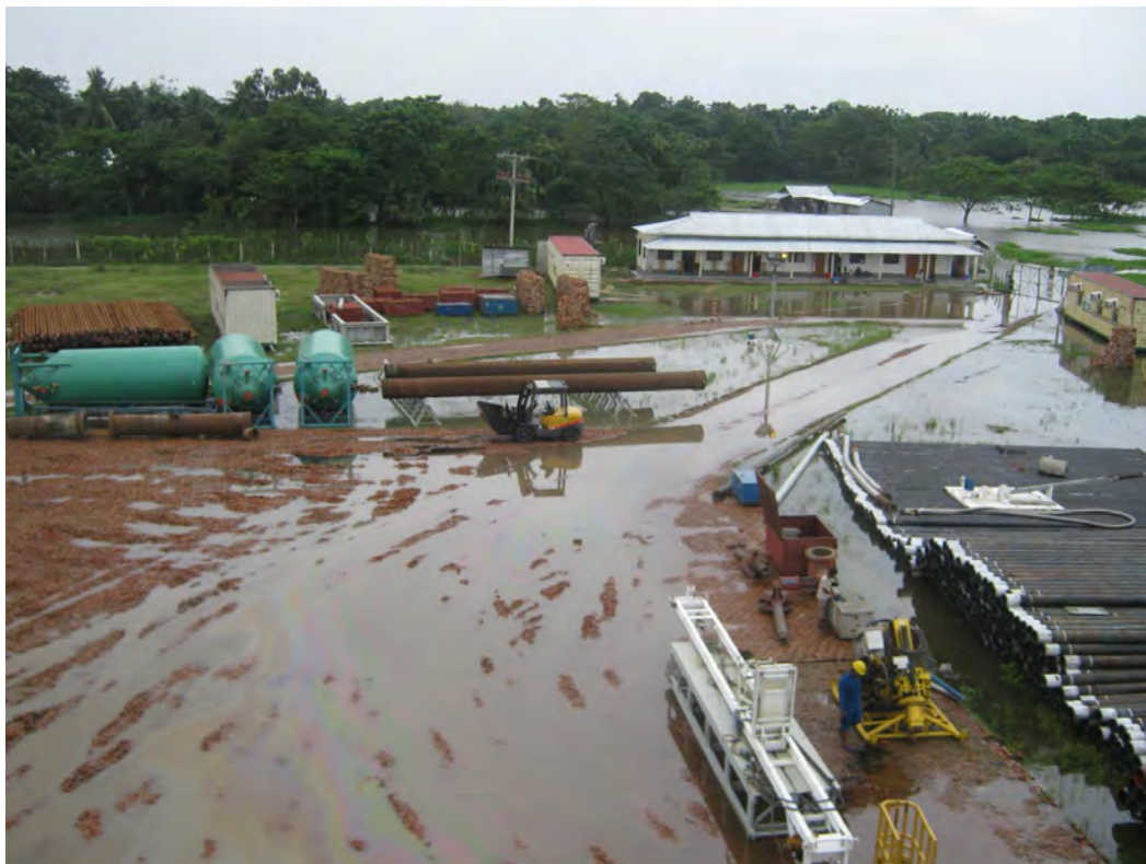
Figure 4.4: Flood water disrupting the drilling in the year 2012 at Sunetra.
