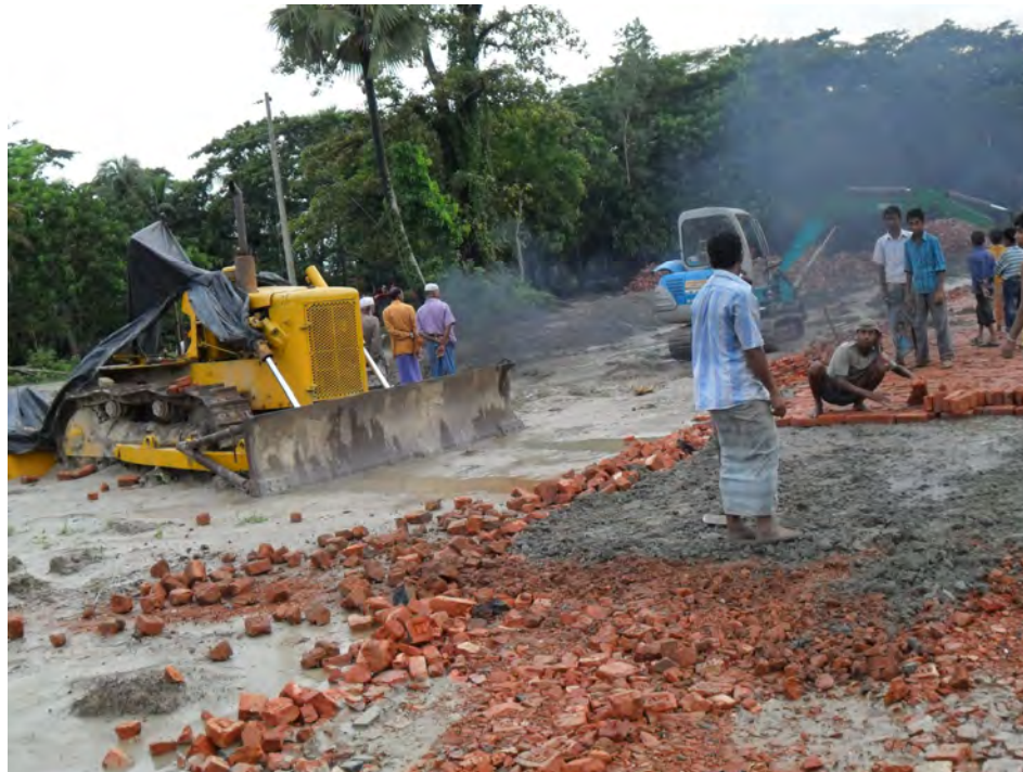
Figure 4.13: Bulldozer used in Sundalpur 1 well site construction.
