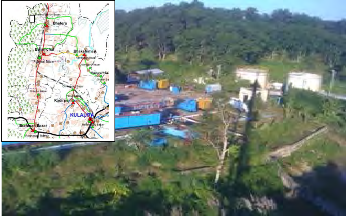
Figure 4.7: Well site scenerio of Vatera 2 (Fenchugonj) gas field, Kulaura, Moulavibazar.
