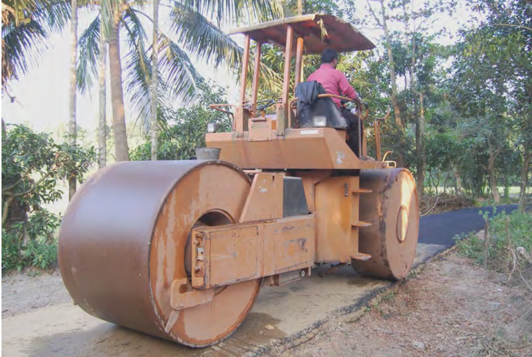
Figure 4.14: Roller used in road at Sundalpur 1 well drilling project.
