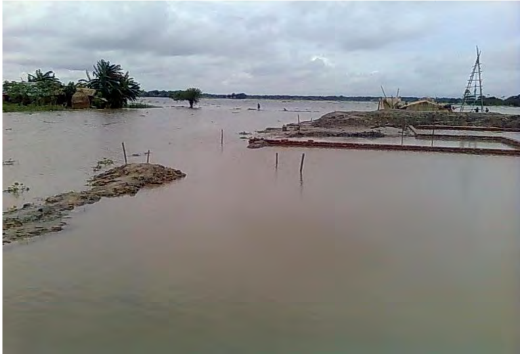
Figure 4.3: Flood water enters the project area and disrupting the communication system in year 2011 at Sunetra.
