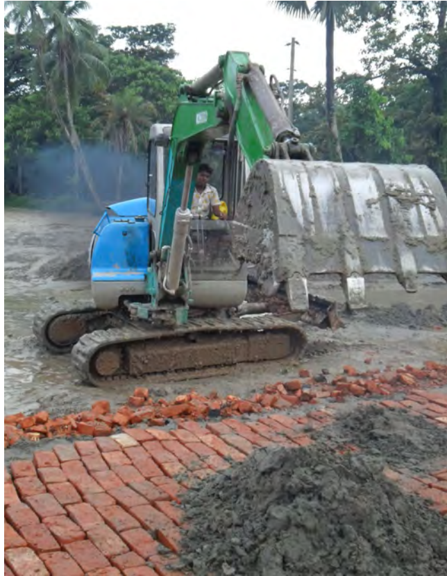
Figure 4.12: Excavator used in Sundalpur 1 well site construction.
