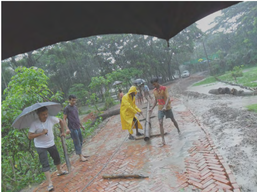
Figure 4.16: Construction works in rain at Sundalpur 1 well drilling project.
