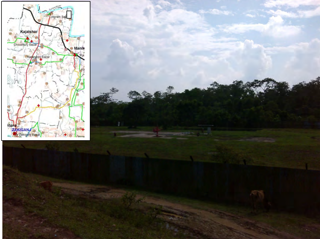
Figure 4.6: Location photograph of Atgram 1 well drilling project.
