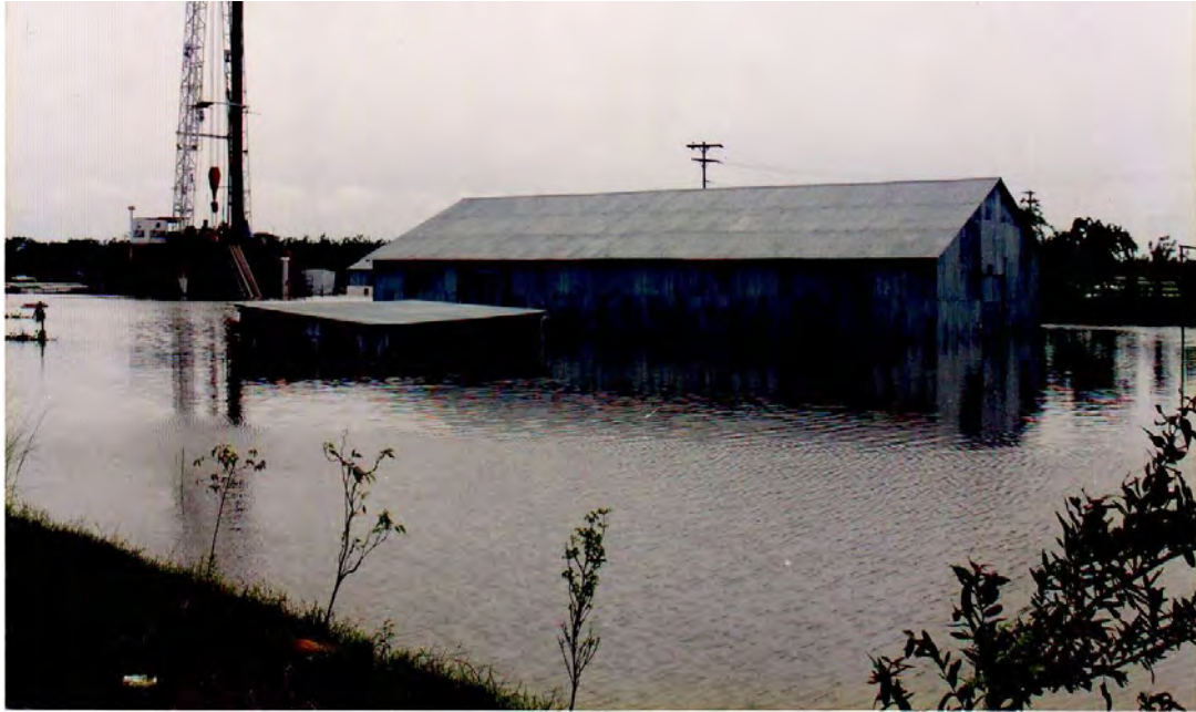
Figure 4.9: Inundation of whole drilling area under flood water at Srikail 1.
