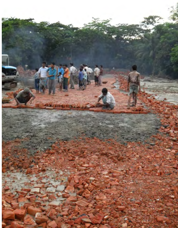
Figure 4.18: Providing brick bats beneath the brick soling of drilling site road.
