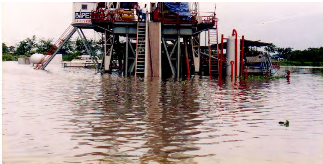
Figure 4.10: Inundation of rig, generator and other infrastructures under flood water at Srikail 1.
