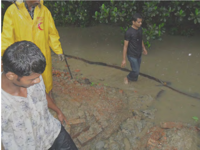
Figure 4.17: Artificial canal/ drain preparation and maintenance to drain out the entrapped water at Sundalpur 1 well drilling project.
