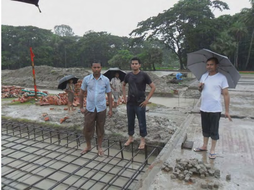
Figure 4.15: Rig foundation construction progresses in rain at Sundalpur 1 well drilling project.
