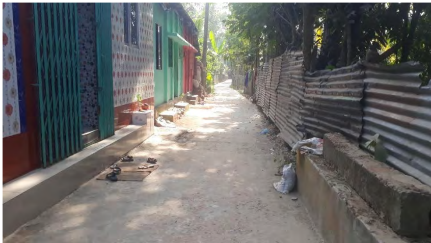
Image C43: RCC drain near Sultan Fokir mazer (south), Bauphal municipality
