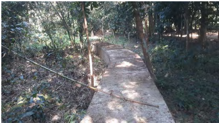
Image C47: Covered RCC drain near Sabanondo, Bauphal municipality
