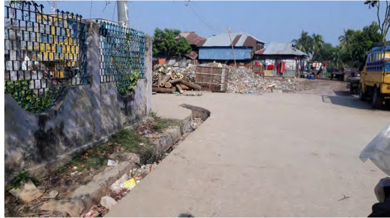
Image C10: Solid waste disposal in the drain in Mongla Port municipality
