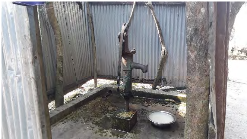
Image C39: Tube well near Satterholader bari (ward 1) in Bauphal municipality
