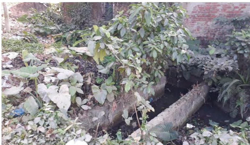
Image C50: Uncovered RCC drain near Poraton Gilrs school, Bauphal municipality
