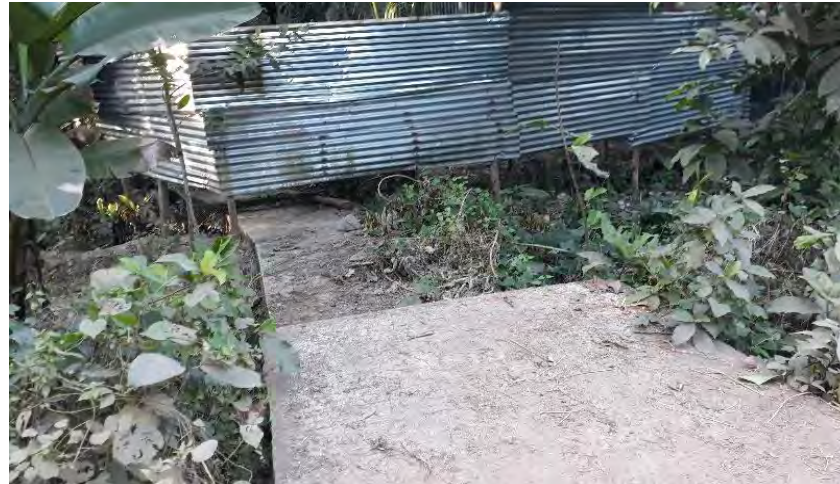
Image C54: Covered RCC drain near Md Waydul mia bari, Bauphal municipality
