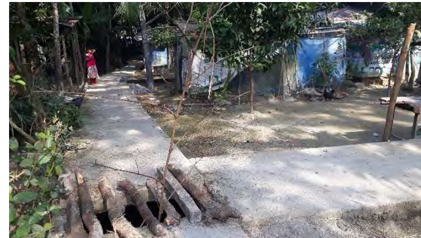
Image C34: RCC drain near Satterholader bari (ward 1) Bauphal municipality
