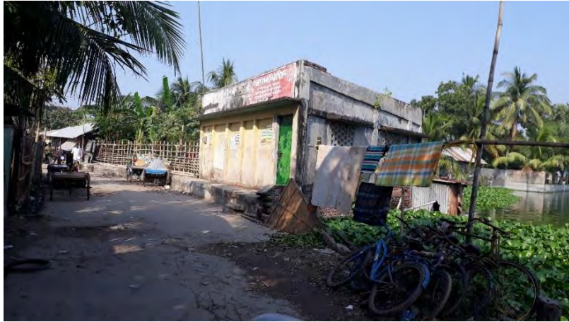
Image C9: RCC drain in Mongla Port municipality
