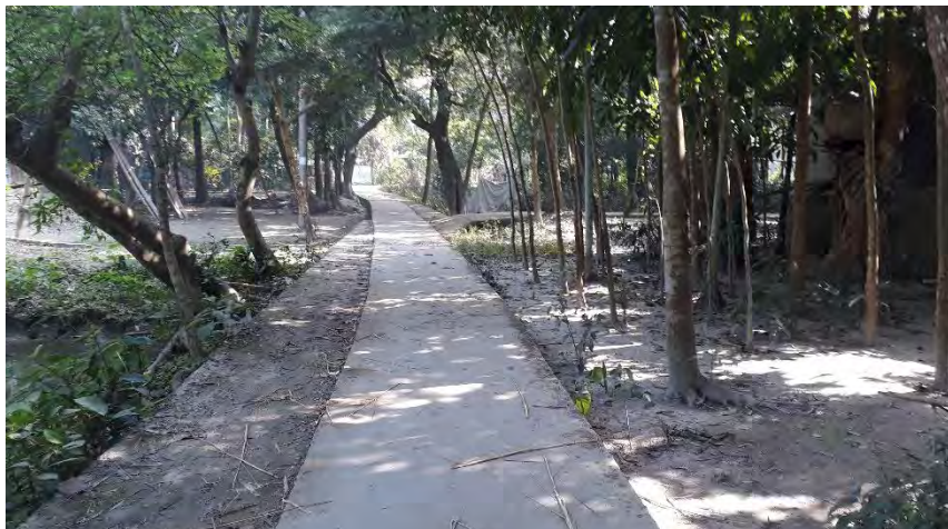
Image C35: RCC drain near Satterholader bari (ward 1) Bauphal
