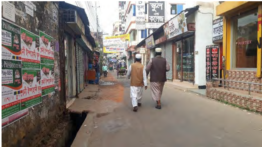
Image C18: RCC drain at Pathanbari road in Feni municipality
