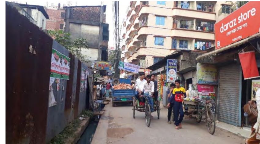
Image C19: RCC drain at Pathanbari road in Feni municipality
