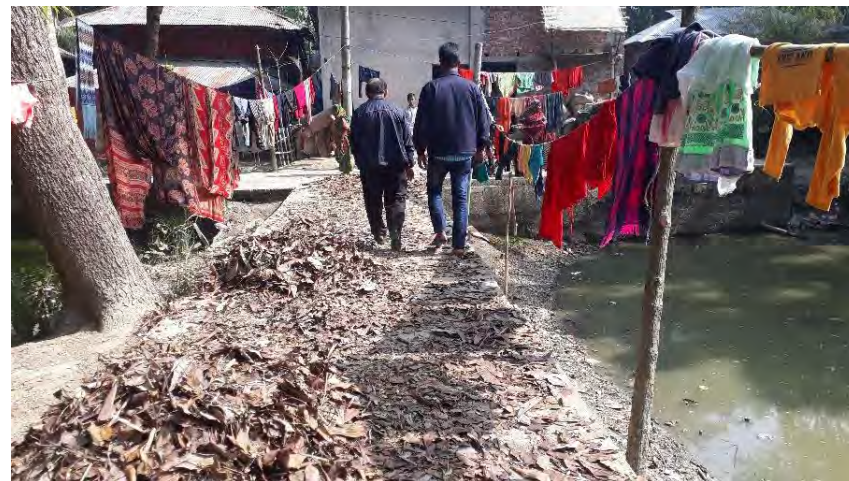
Image C36: RCC drain near Satterholader bari (ward 1) Bauphal municipality
