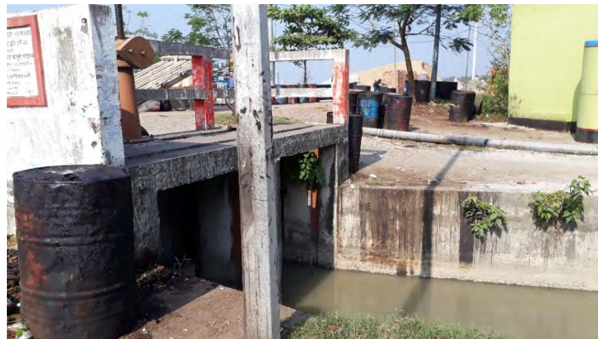
Image C11: Sluice gate near Thakurain Khal in Mongla Port municipality
