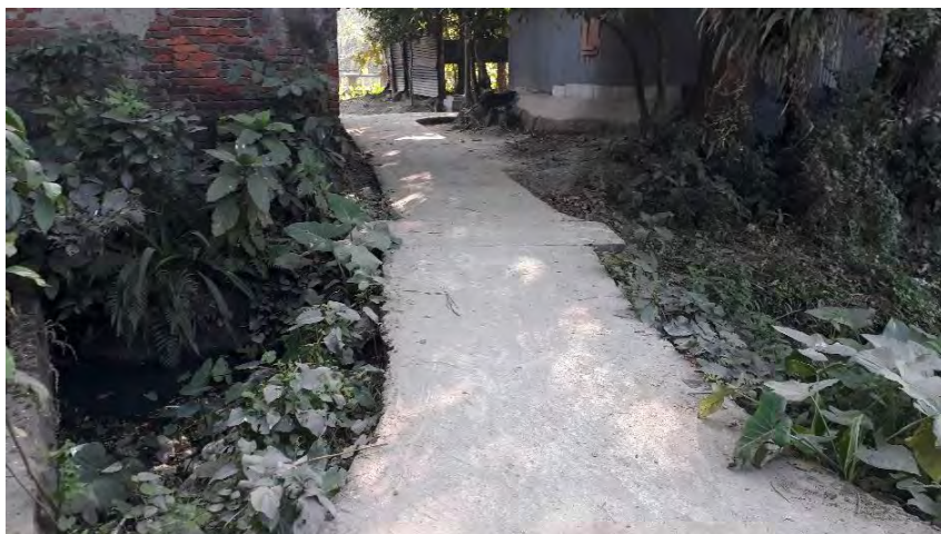
Image C49: Covered RCC drain near Poraton Gilrs school, Bauphal municipality
