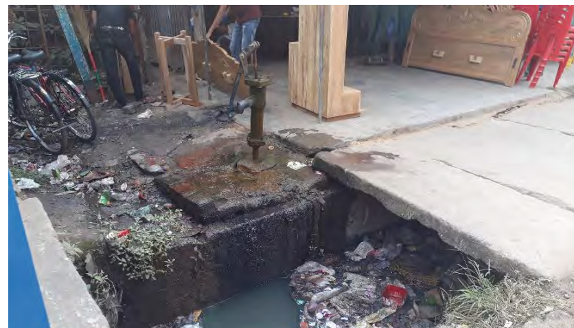
Image C32: Solid waste dumping at RCC drain near Mohipal in Feni municipality
