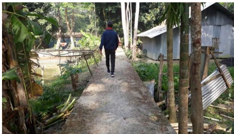
Image C40: RCC drain near Nitaipalli bari Bauphal municipality
