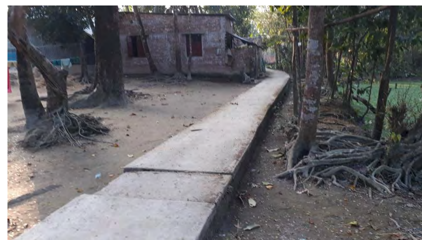
Image C58: Covered RCC drain near Sarderbari to sadhu howlader bari, Bauphal municipality
