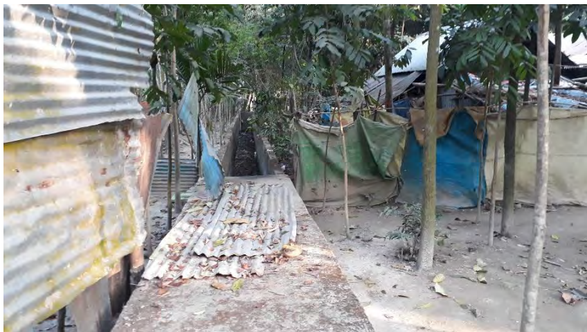
Image C55: RCC drain near Forkania madrasa, Bauphal municipality
