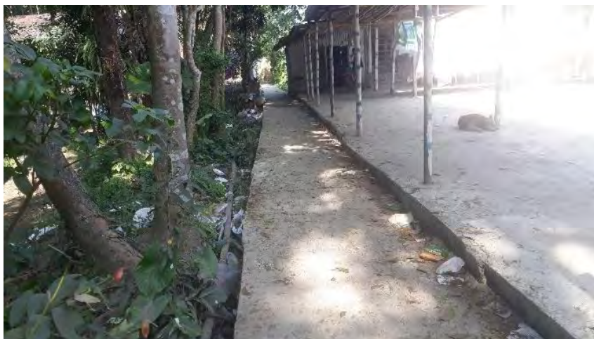
Image C45: Covered RCC drain near Md Nazrul islam bari, Bauphal municipality
