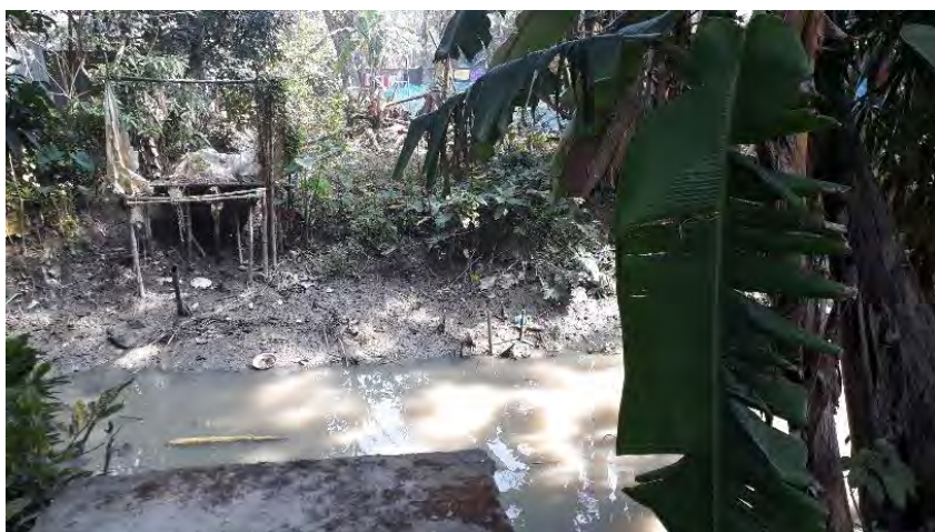
Image C37: Discharge point of the RCC drain near Satterholader bari (ward 1) in Bauphal municipality
