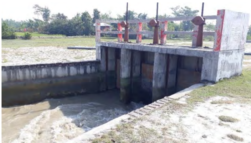
Image C5: Sluice gate near the embankment in Mongla Port municipality
