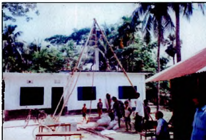
Photograph-11: Deep Drilling Point
