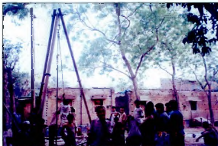
Photograph-12: Deep Drilling Working
