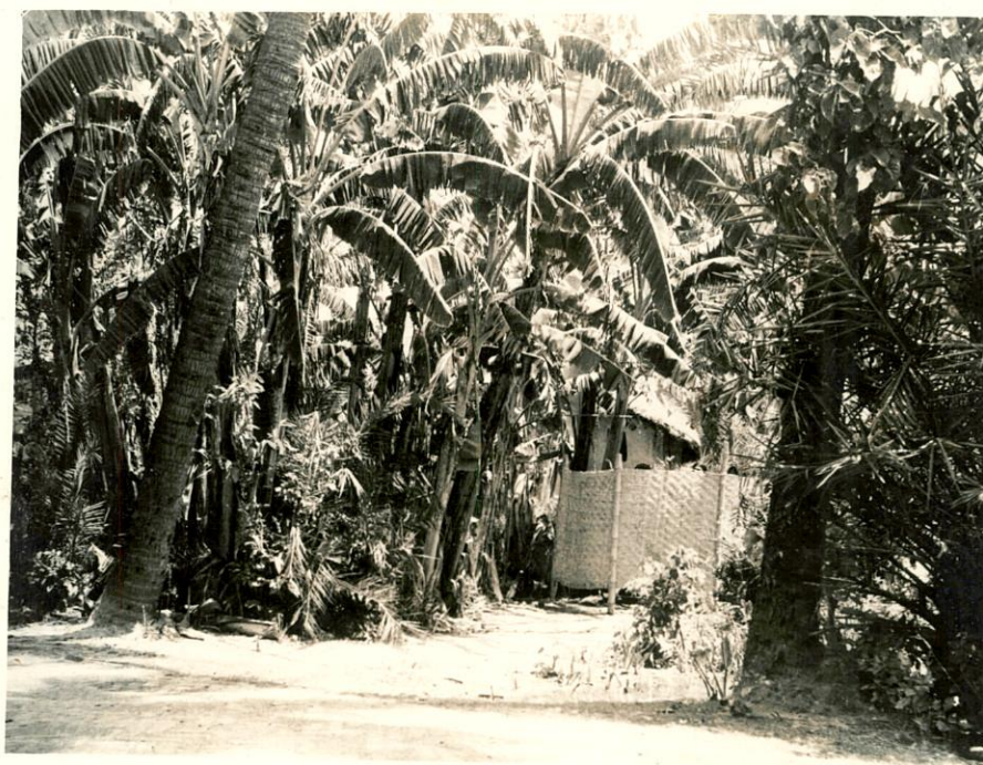
Plate-16 Arrangement for partial privacy at tubewell site by constructing tarza fencing.
