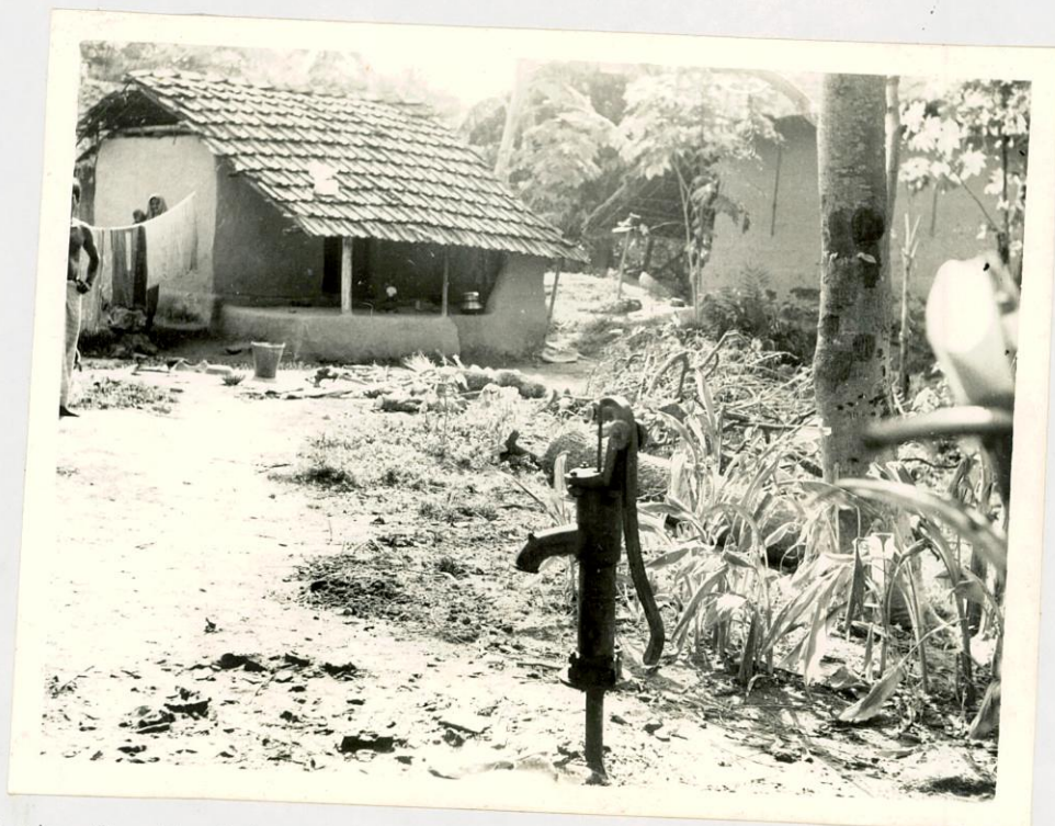
Plate-9 Washing and bathing is very difficult at tubewell site where there is no platform.
