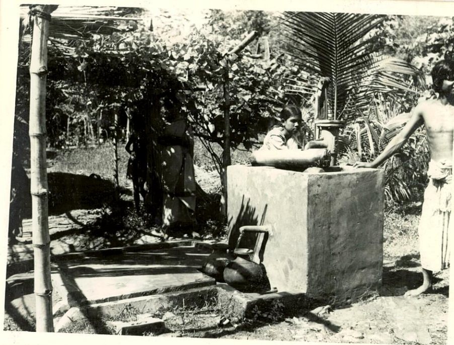
Plate-6 Iron removal plant No. 1.
