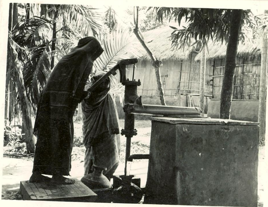
Plate-7 Iron removal plant No. 2.
