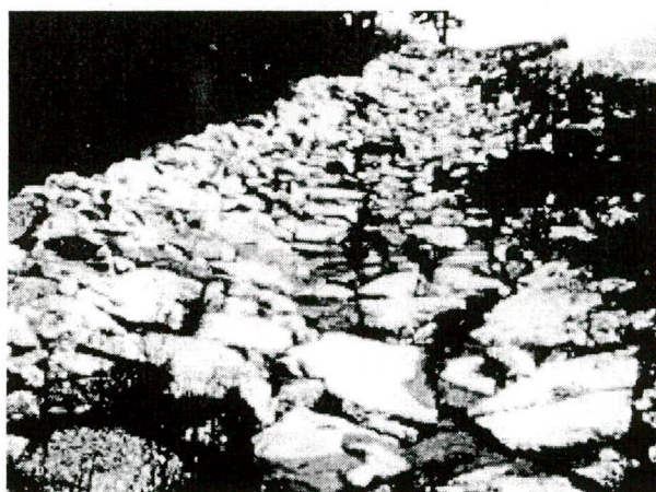
Figure 2.4: Broken Concrete Riprap (Source: Brown and Clyde, 1989)
