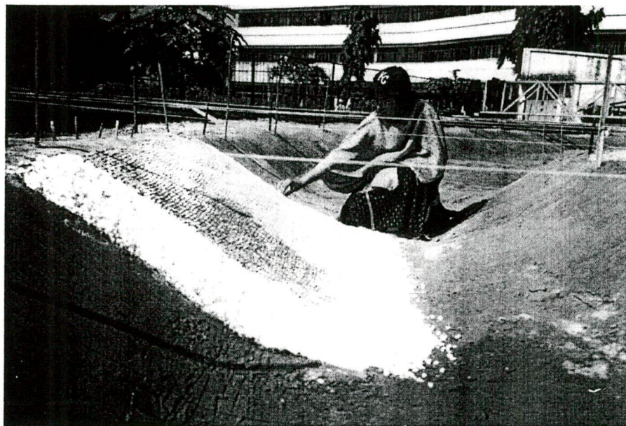
Photograph C.13 Placing blocks on the slope of bank protection
