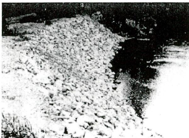
Figure 2.2 Hand-placed Riprap (Source: Brown and Clyde, 1989)
