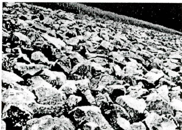
Figure 2.1 Dumped Rock Riprap (Source: Brown and Clyde, 1989)
