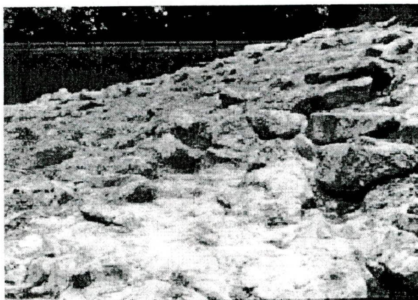
Figure 2.8 Grouted Rock (Source: Brown and Clyde, 1989)
