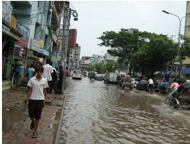
Fig: 4.4 Poor and Dilapidated footpaths and roads
