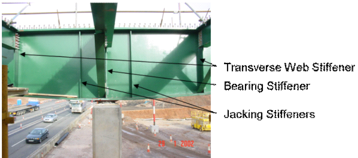
Figure 1.4: Transverse web stiffeners.
