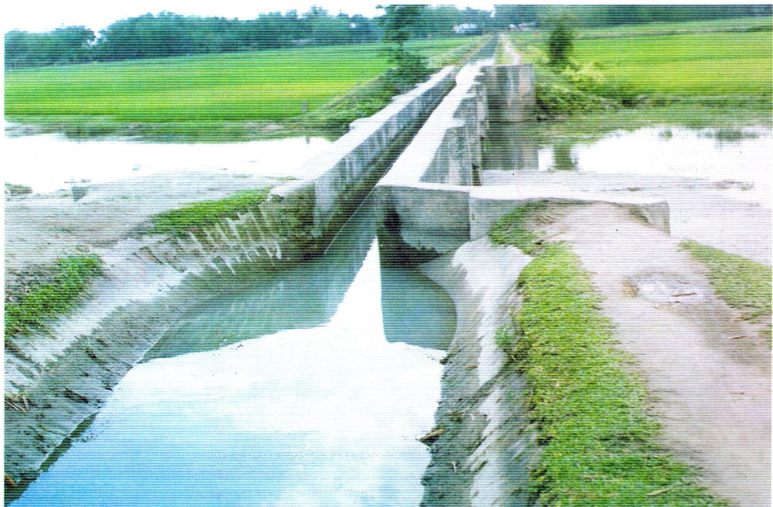
Figure 1.8 Convey water over drainage Khal
