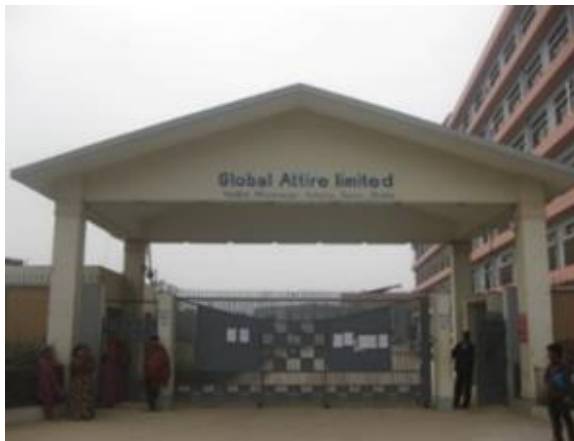
Figure 3.12: Front side of the case RMG building
