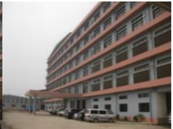
Figure 3.13: South elevation of the case RMG building
