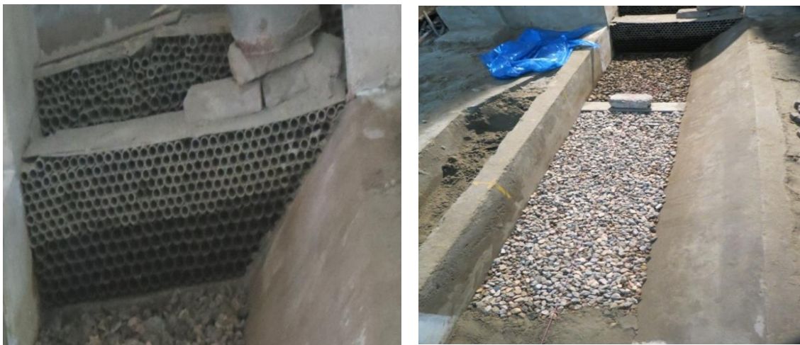
Figure 4.5: Diffuser pipes and upstream stone bed
