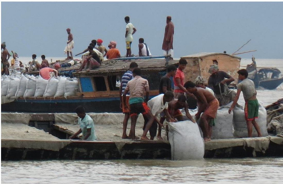
Figure 2.4: Geobags dumping at Sirajgonj Hard Point (Field visit on 15.08.2013)
