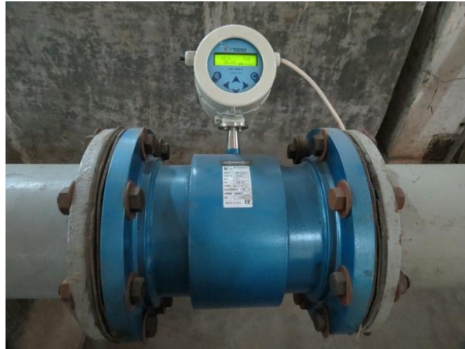
Figure 4.12: Flow meter
