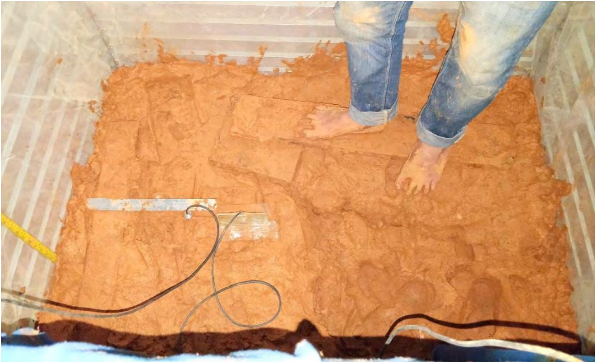
Figure 4.10: Placement of third layer of clayey soil.
