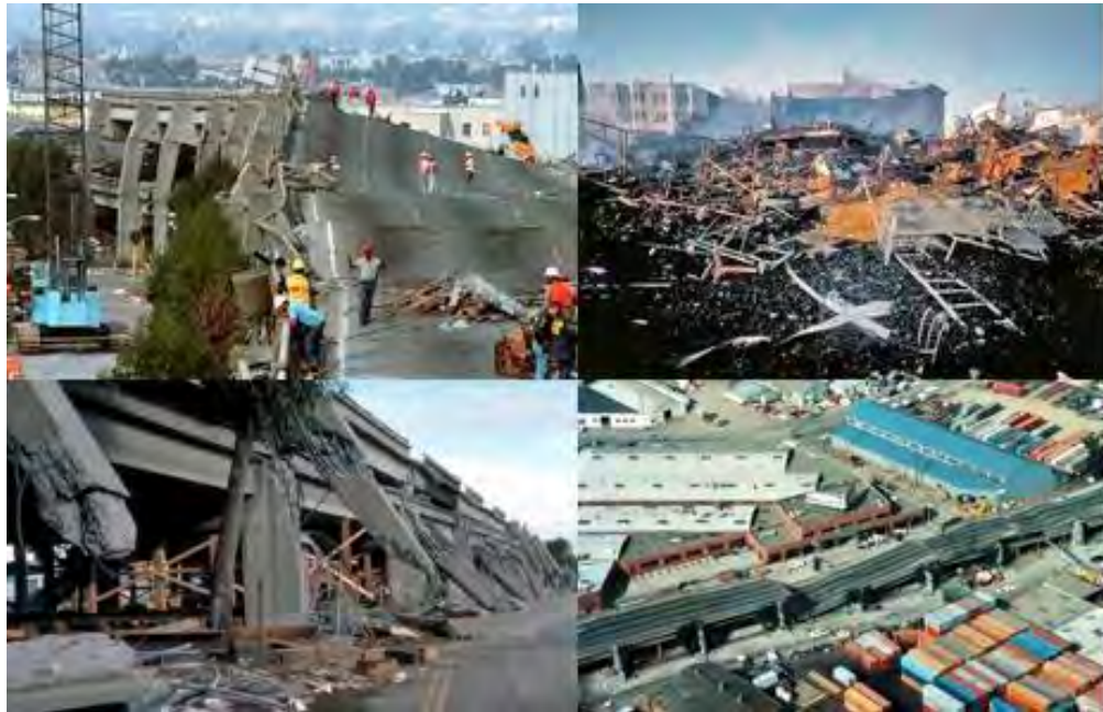
Figure 2.7 : Damage of different infrastructures due to Loma earthquake
