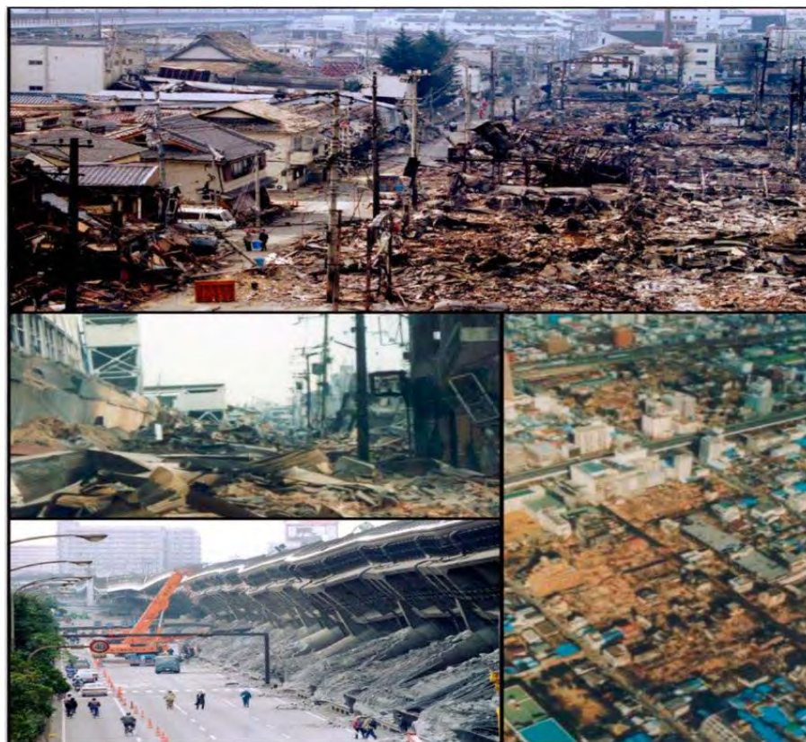
Figure 2.6: Damage of different infrastructures due to Kobe earthquake
