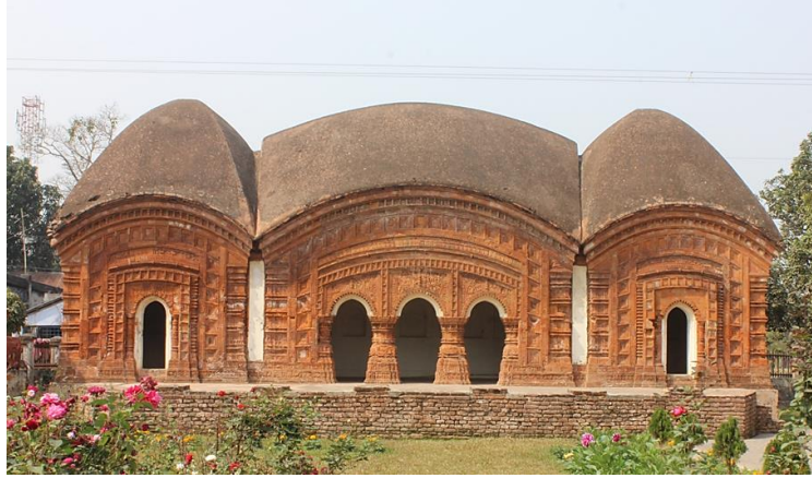
(a) East façade of the Temple
