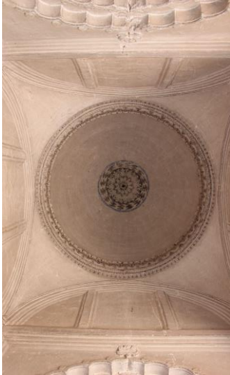
The inner side of the roof , Corner open veranda
