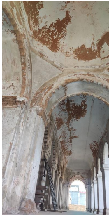
(b) Inner roof of corner
