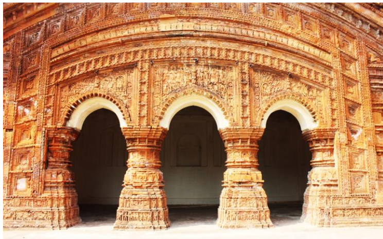
(b) East façade of the main Sanctum in the middle
