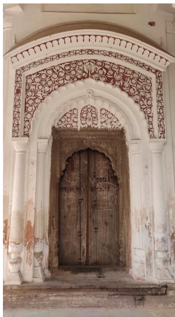
(c) Entrance Door to Garbhagriha or main sanctum Source: Author's Collection; Site Survey
