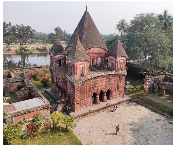
Figure 49 : View from the Inner Panch Ani Palace Source: Author's Collection; Site Survey
