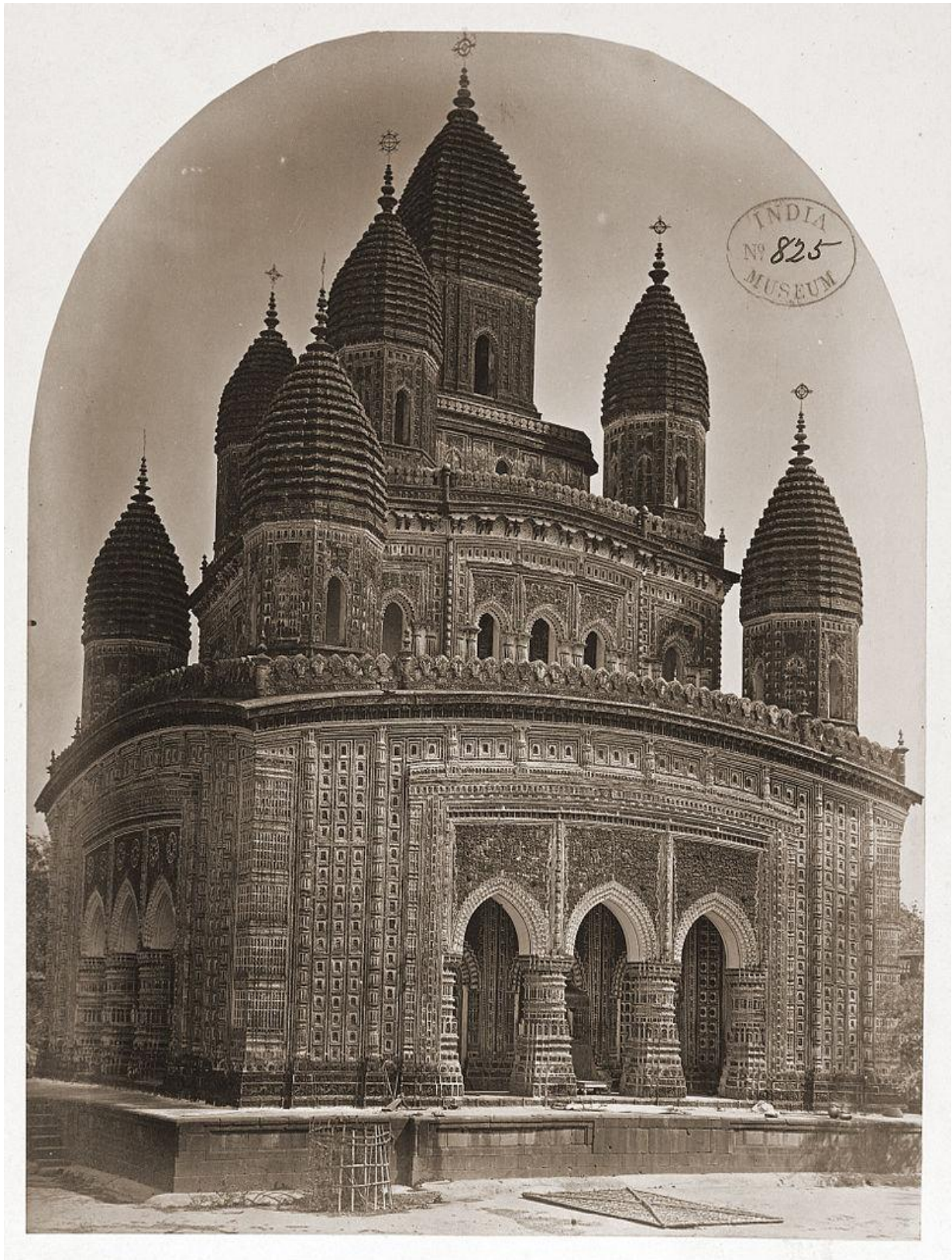
Figure 19 : A southern view of Kantojiu Temple in 1871 shows the nine spires that were subsequently destroyed in an earthquake
