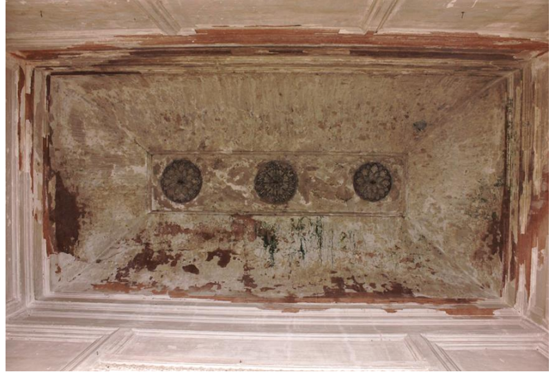
The inner side of the roof, Middle Open Veranda
