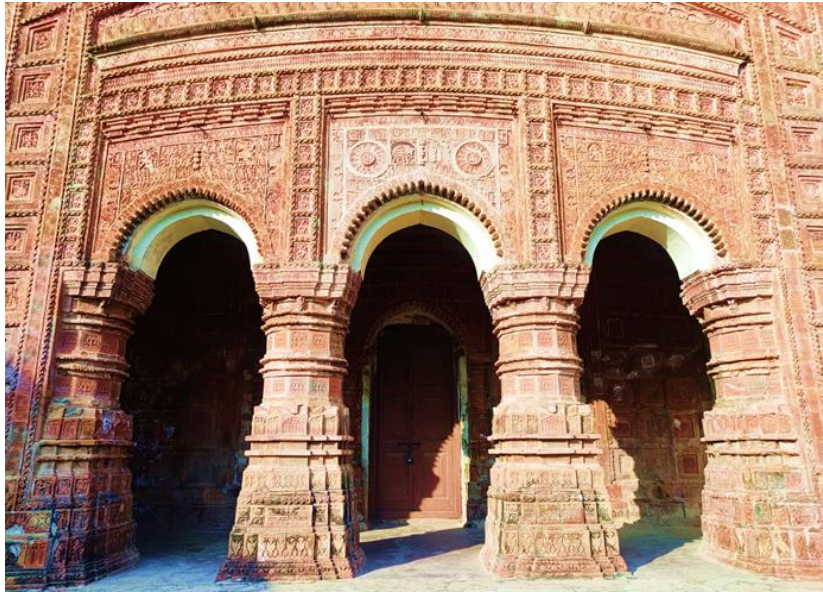
(a) Terracotta details of South facade
