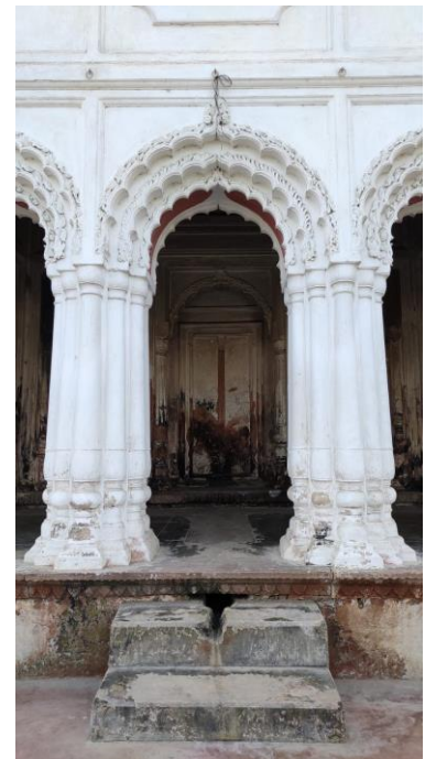
Water Drainage from main sanctum
