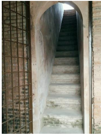
Stair on the West
