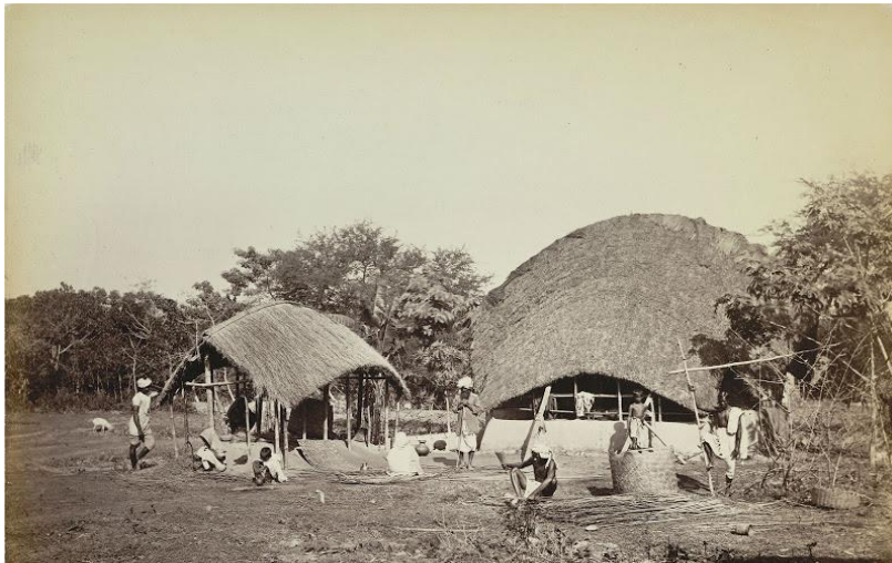
these hut roofs were built curved to throw off the heavy monsoon rain more effectively using the flexibility of bamboo
