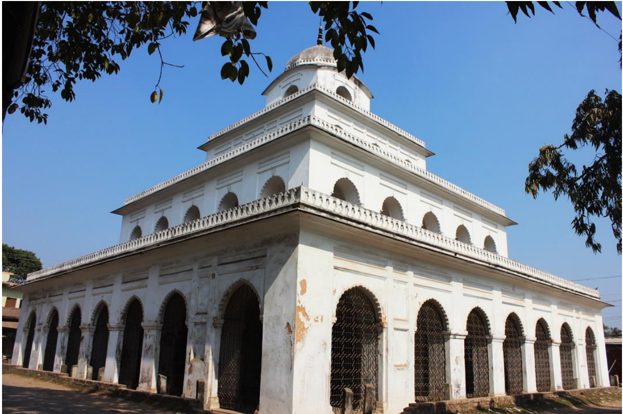
View from front Road side
