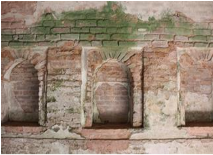
(a) Interior North Wall
