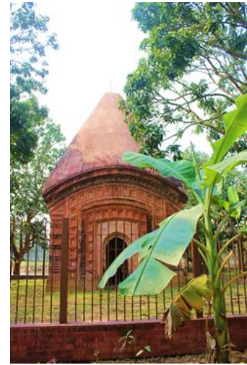
(b) East Facade
