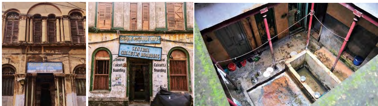
Figure 3.1: Old mess houses in India.
