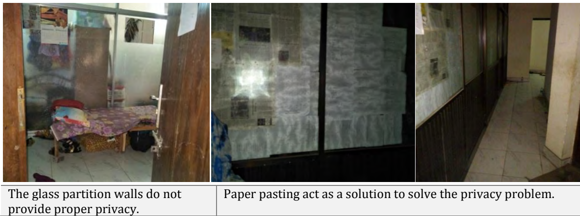
Figure 6.12: the situation of a glass partitioned wall.
