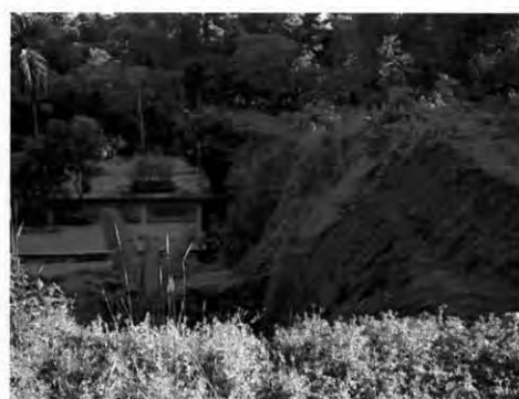
Nurani, Landslide Hazard
